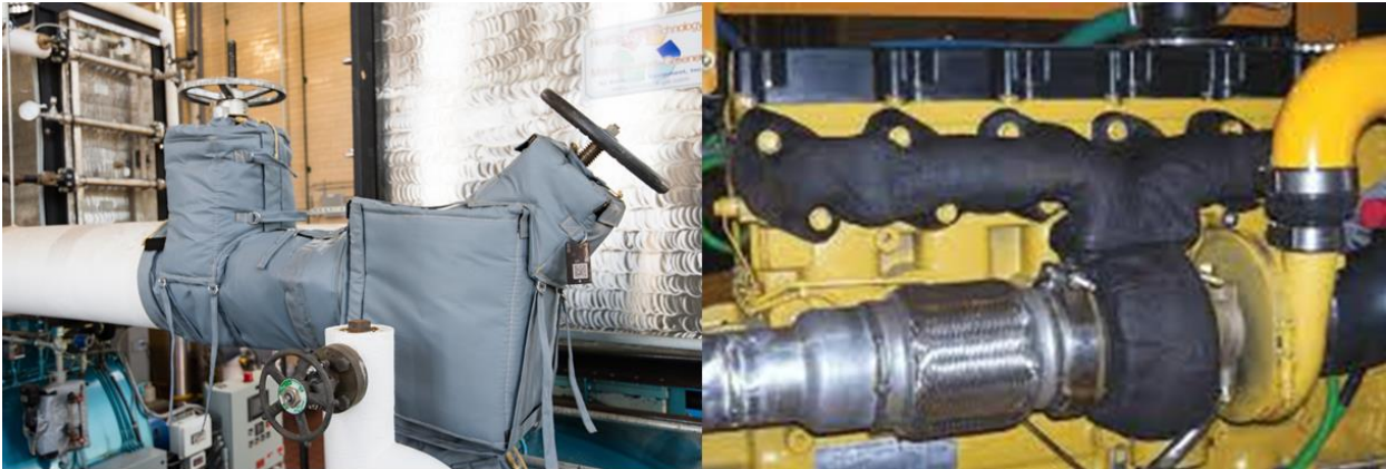
Figure 3 – HTIW blankets covering balance of plant components (left) [9] and an exhaust manifold of a large ICE (right) [10].
